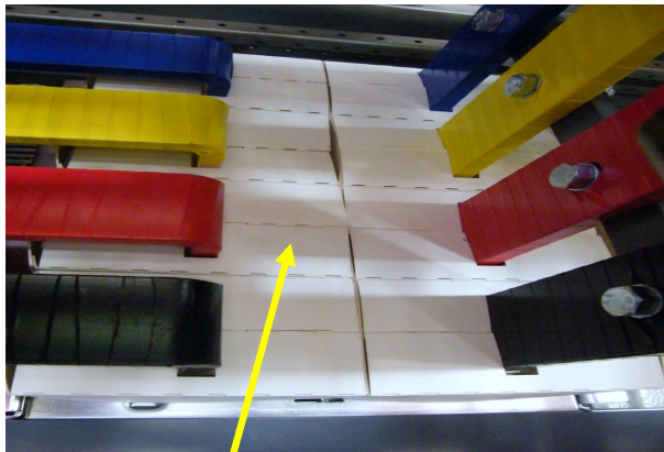
Position of Formex in busbar application
